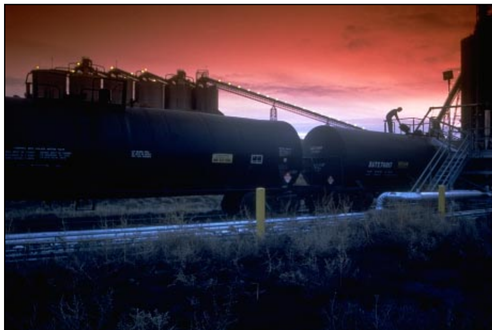
Tank car loading facility for Coal Derived Liquid at ENCOAL demonstration plant.
