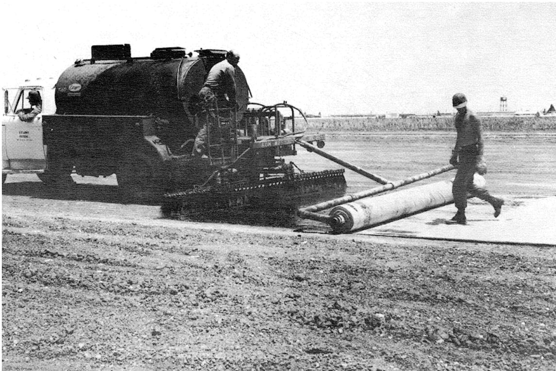
Figure 3-2. Rolling frame for placing polypropylene fabric over the first coat of asphalt emulsion.
